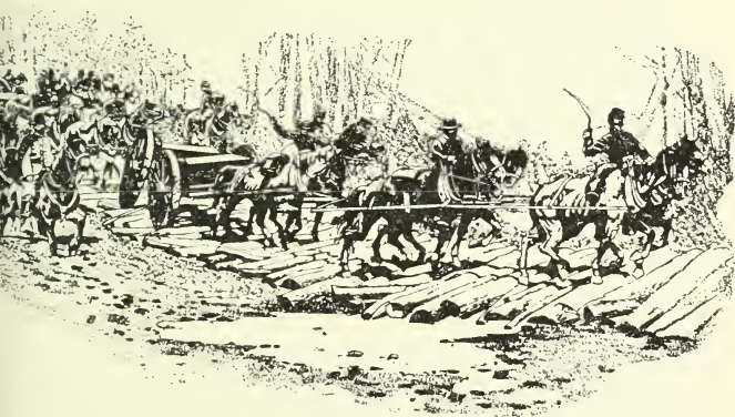
Corduroy Road—All Hand-labor
